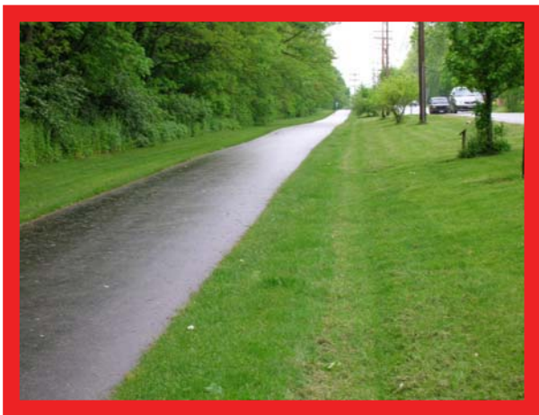
Land Use Figure 21. Corry Street features a dedicated bikeway parallel to the roadway Source: Justin Milam
