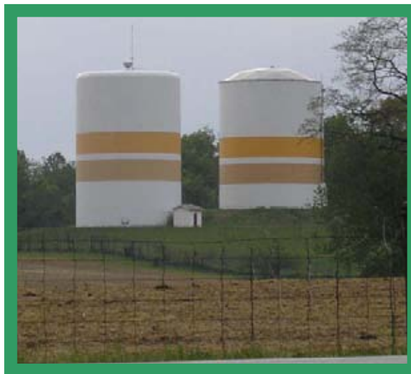
Energy Figure 11. Yellow Springs' water towers Source: Tim Burgener
