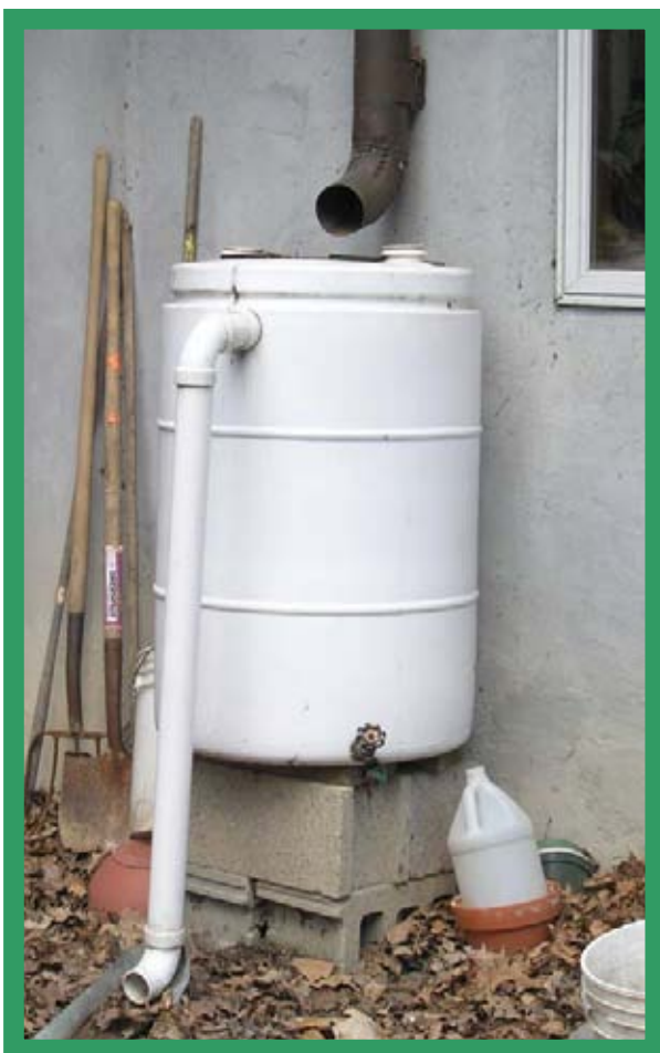
Energy Figure 18. This barrel at a local residence collects rainwater from the downspout for reuse Source: Tim Burgener
