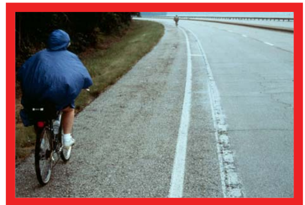
Land Use Figure 26. Paved shoulders enable safe bicycling in areas with lower cycling demand Source: Ped Bike Images
