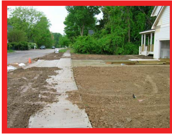
Land Use Figure 27. Subdivision regulations should require 5-foot sidewalks instead of 4-feet, as shown here Source: Justin Milam
