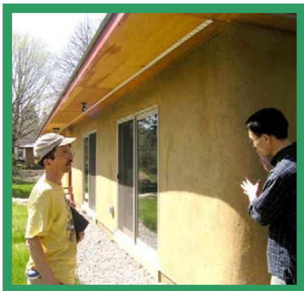
Energy Figure 2. Andy Holyoke (left) describing the local materials used for this straw-bale house Source: Tim Burgener
