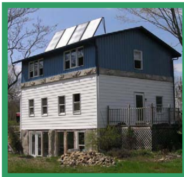
Energy Figure 3. Solar collectors added during a remodel of an older home Source: Tim Burgener
