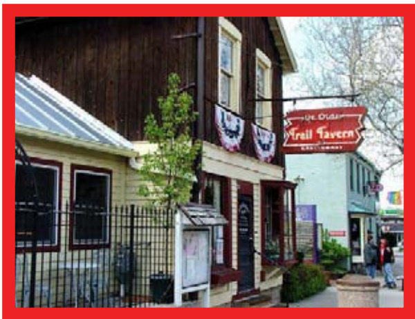
Land Use Figure 15. Yellow Springs' Historic Ye Old Trail Tavern Source: Urban Ohio
